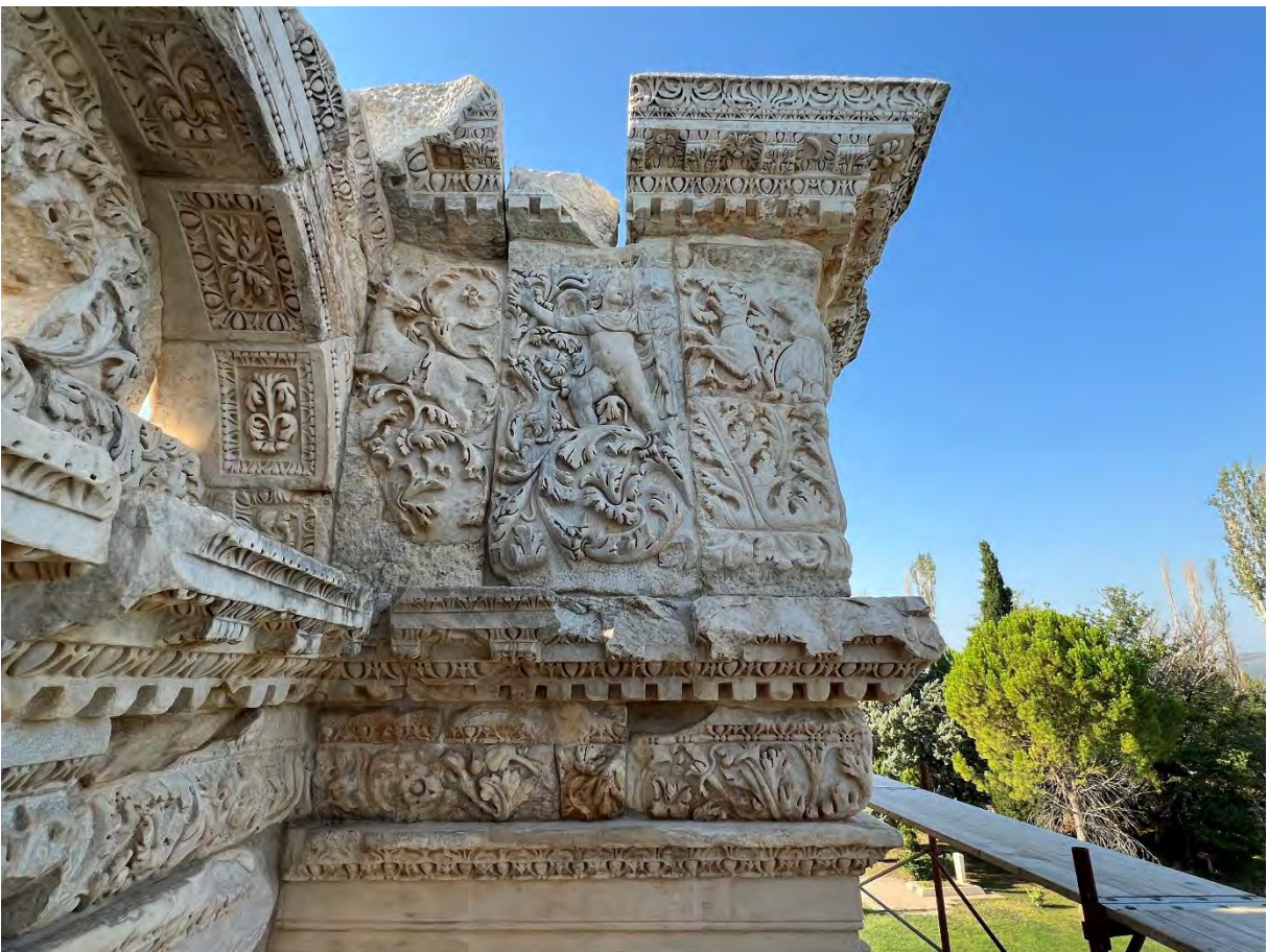
Figure 49: Tetrapylon. West side. Anastylis of carved marble facade cleaned and conserved, looking south (2024).
