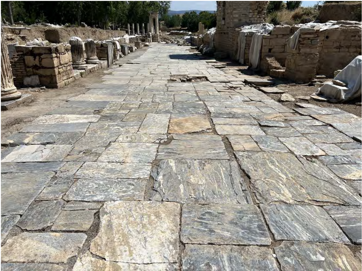
Figure 51: Tetracylon Street. Looking south towards Sebasteion Propylon, showing restored blue-grey marble street paving (2024).
