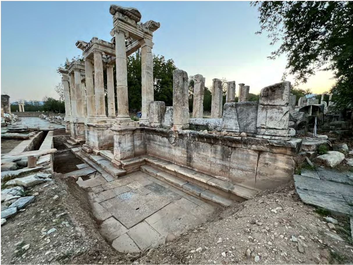
Figure 52: Tetrapylon Street. Looking north, showing restored walls of late antique street drain at left in front of Sebasteion Propylon and exposed area of original 1st-century paving in centre foreground (2024).
