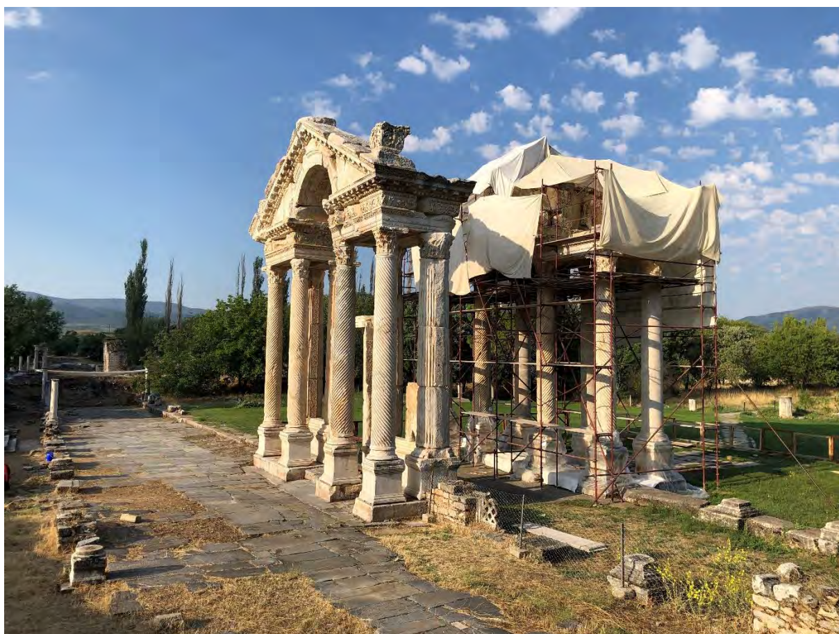
Figure 47: Tetrapylon. West side of anastylosis scaffolded for conservation and maintenance (2024).
