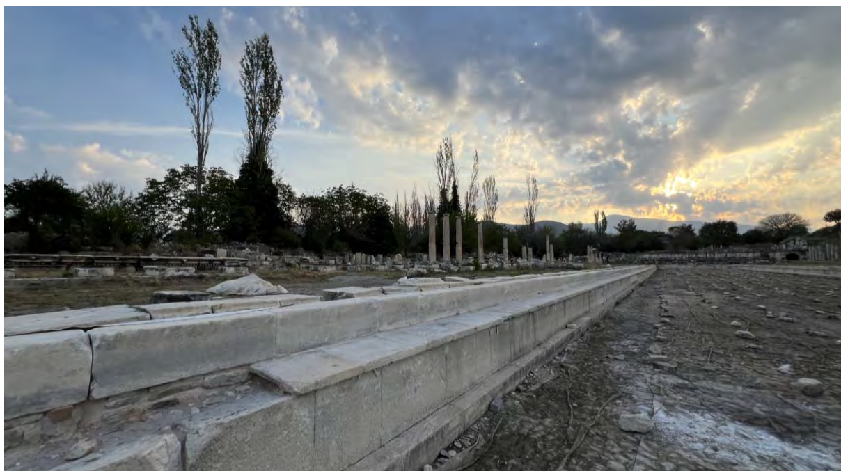
Figure 46: Place of Palms. Conservation of north side of pool's marble perimeter (2024).
