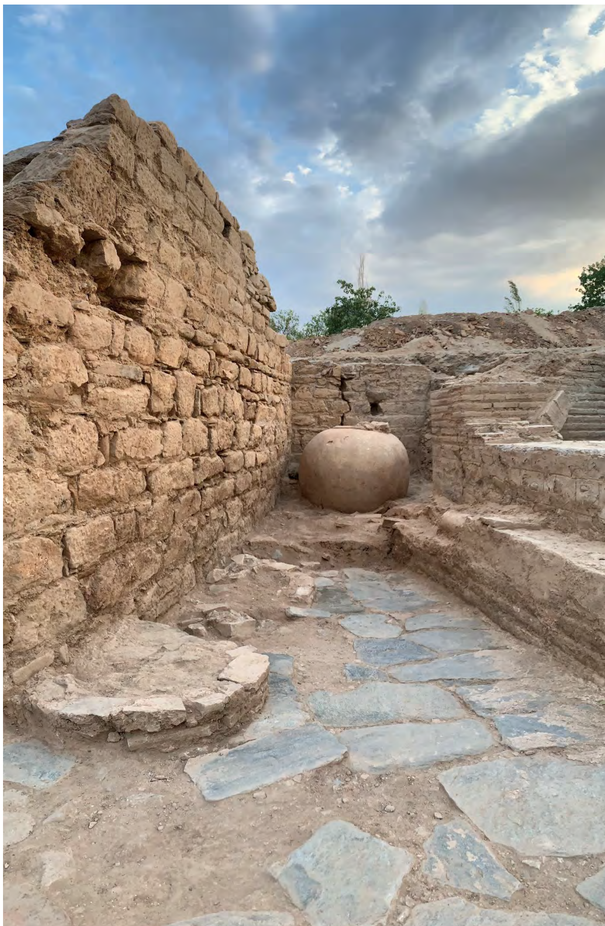
Figure 17: House of Kybele. Western arm of corridor around apse (Room 10), looking south, with remains of built supports for storage vessels at left, stone pithos at far end, and waterpipe visible at right (2024).
