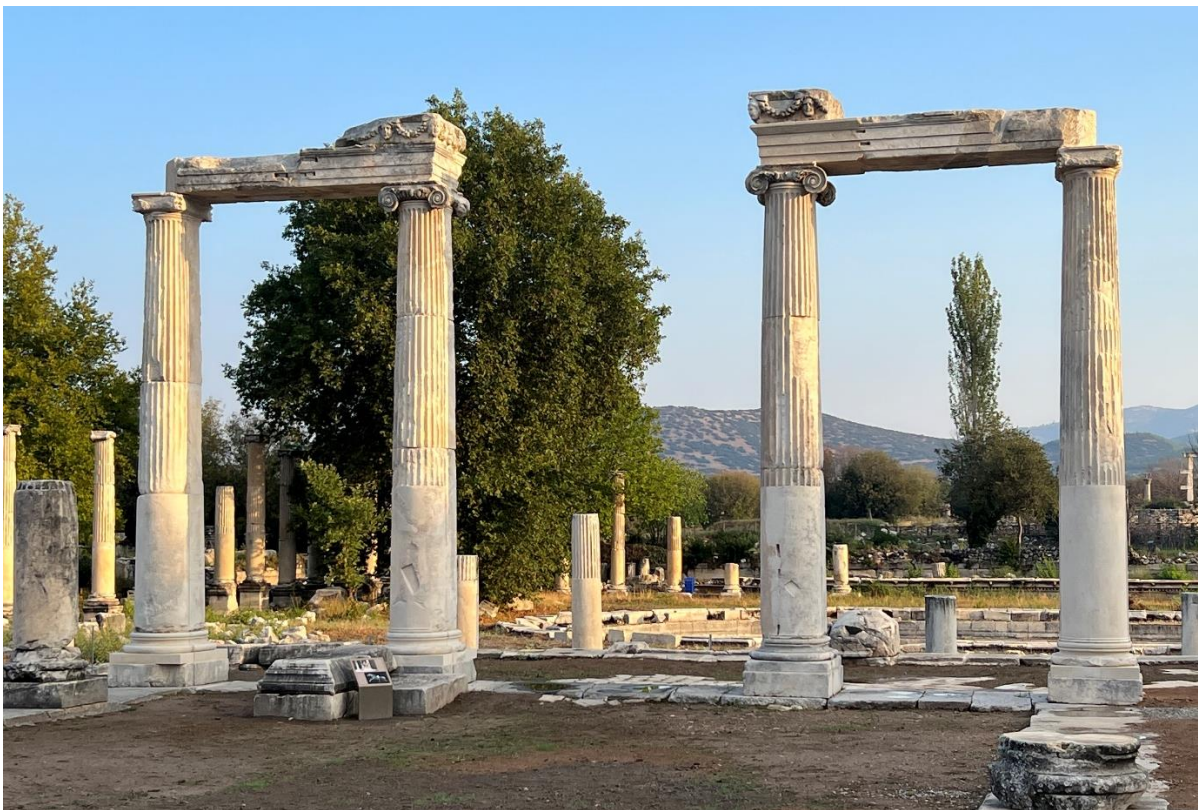
Figure 12: Civil Basilica. Completed anastylosis of colossal columnar order of vestibule (2023).
