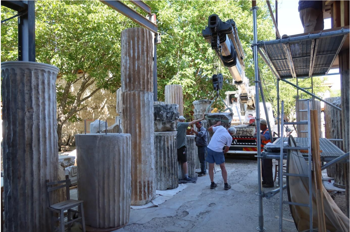
Figure 9: Civil Basilica. Study for anastylosis of colossal columns from vestibule of Basilica in depot-workshop (2023).
