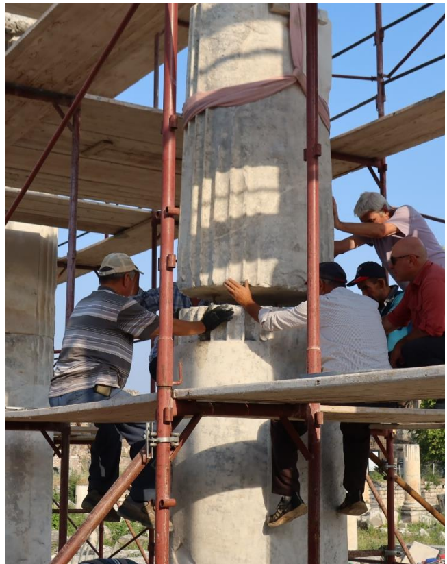
Figure 10A-B: Civil Basilica. Anastylosis work in progress on colossal double half-columns of vestibule (2023).
