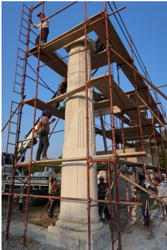
Figure 10A-B: Civil Basilica. Anastylosis work in progress on colossal double half-columns of vestibule (2023).
