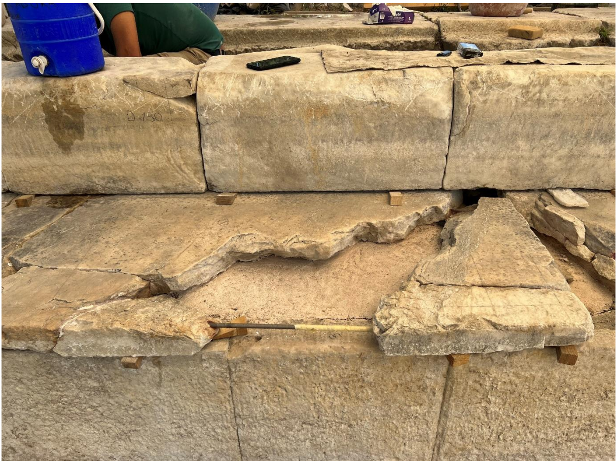
Figure 14: Place of Palms. Conservation of pool's northern marble perimeter, detail of shattered inner foot-plate (2023).
