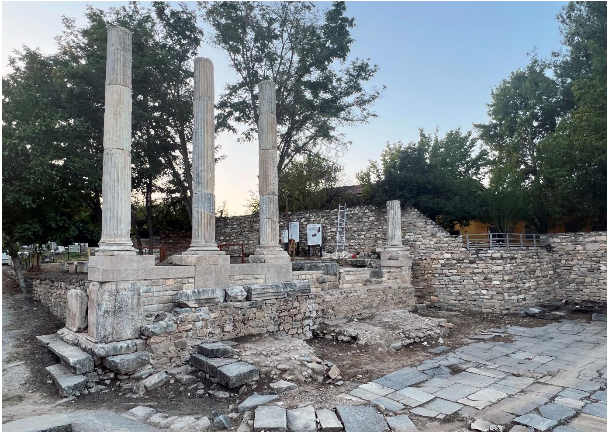
Figure 42: Sebasteion Temple. Anastylosis of columns of temple façade (2023).
