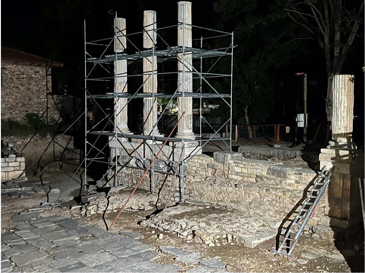
Figure 41: Sebasteion Temple. Anastylosis of columns of temple façade (2023).
