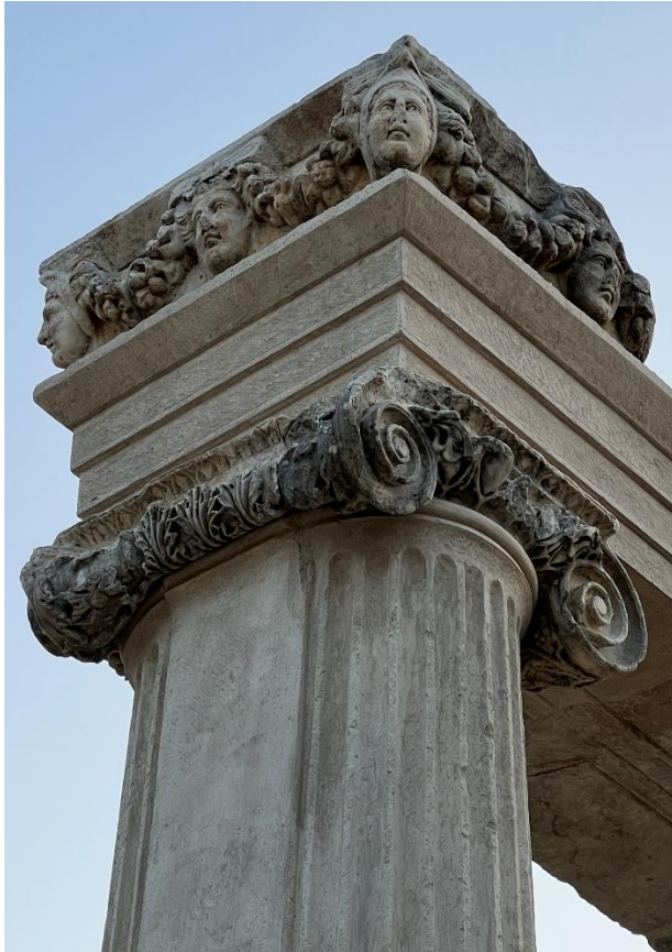
Figure 11A-B: Civil Basilica. Anastylosis of colossal marble order of vestibule (2023).
