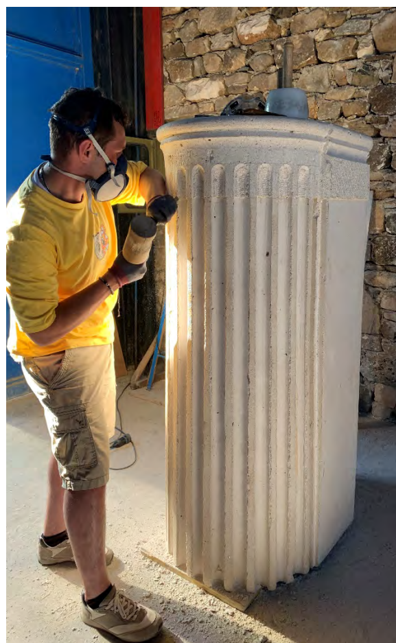
Figure 9A–B: Civil Basilica. A: Joining broken architrave. B: Hand-working flutes of replacement column drum (2022).
