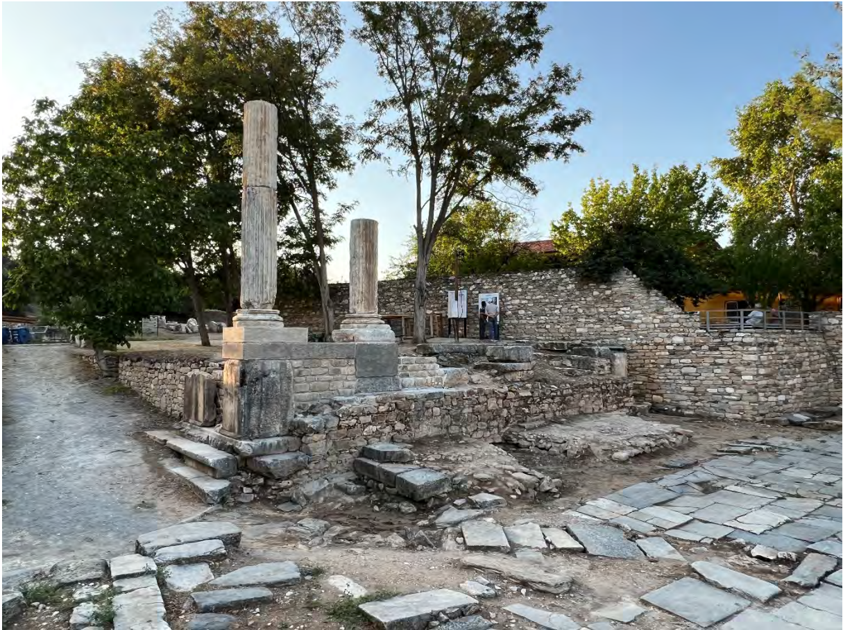
Figure 44: Sebasteion Temple. Anastylosis of parts of two columns, looking south-east at end of 2022.
