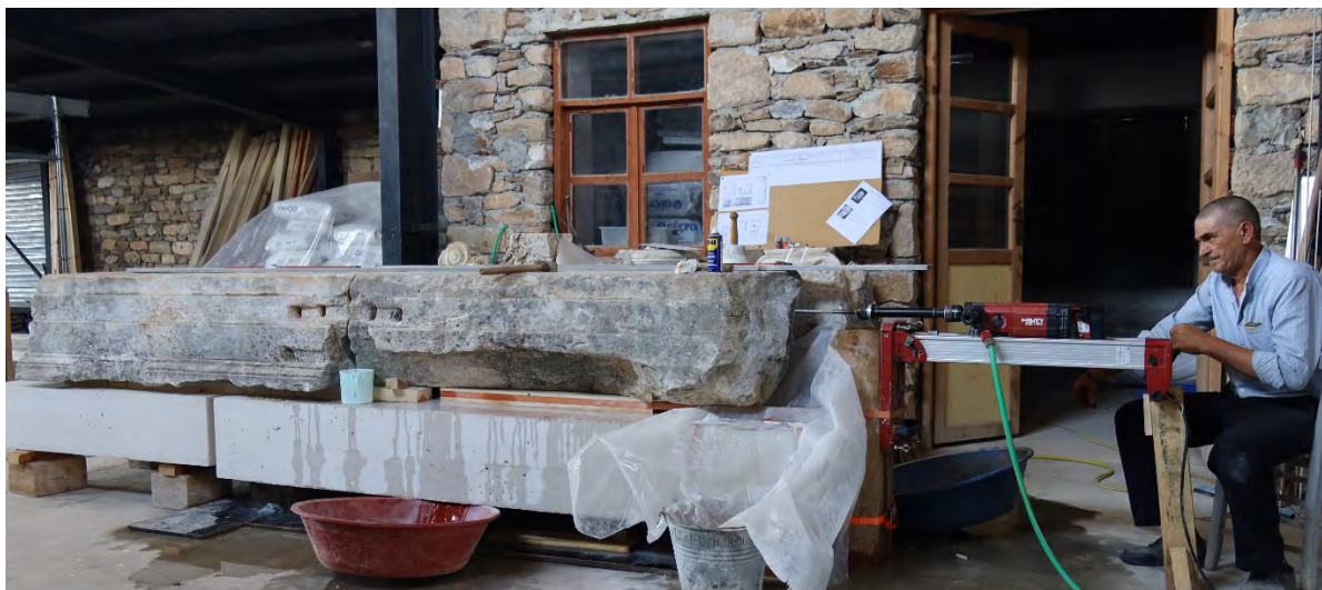
Figure 8: Civil Basilica. Drilling of four-metre-long architrave, already broken and repaired with clamps in antiquity (2022).
