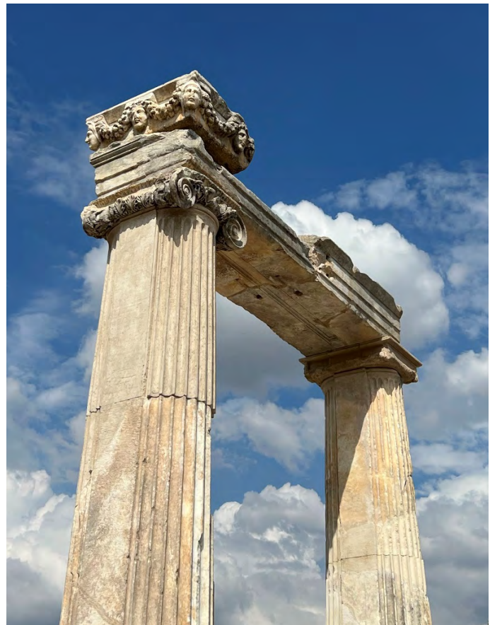
Figure 13A–B: Civil Basilica. A: Fitting of Ionic capital. B: Architrave in position, with frieze block on top (2022).
