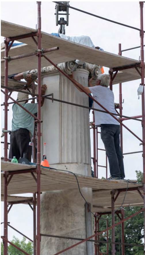
Figure 13A–B: Civil Basilica. A: Fitting of Ionic capital. B: Architrave in position, with frieze block on top (2022).
