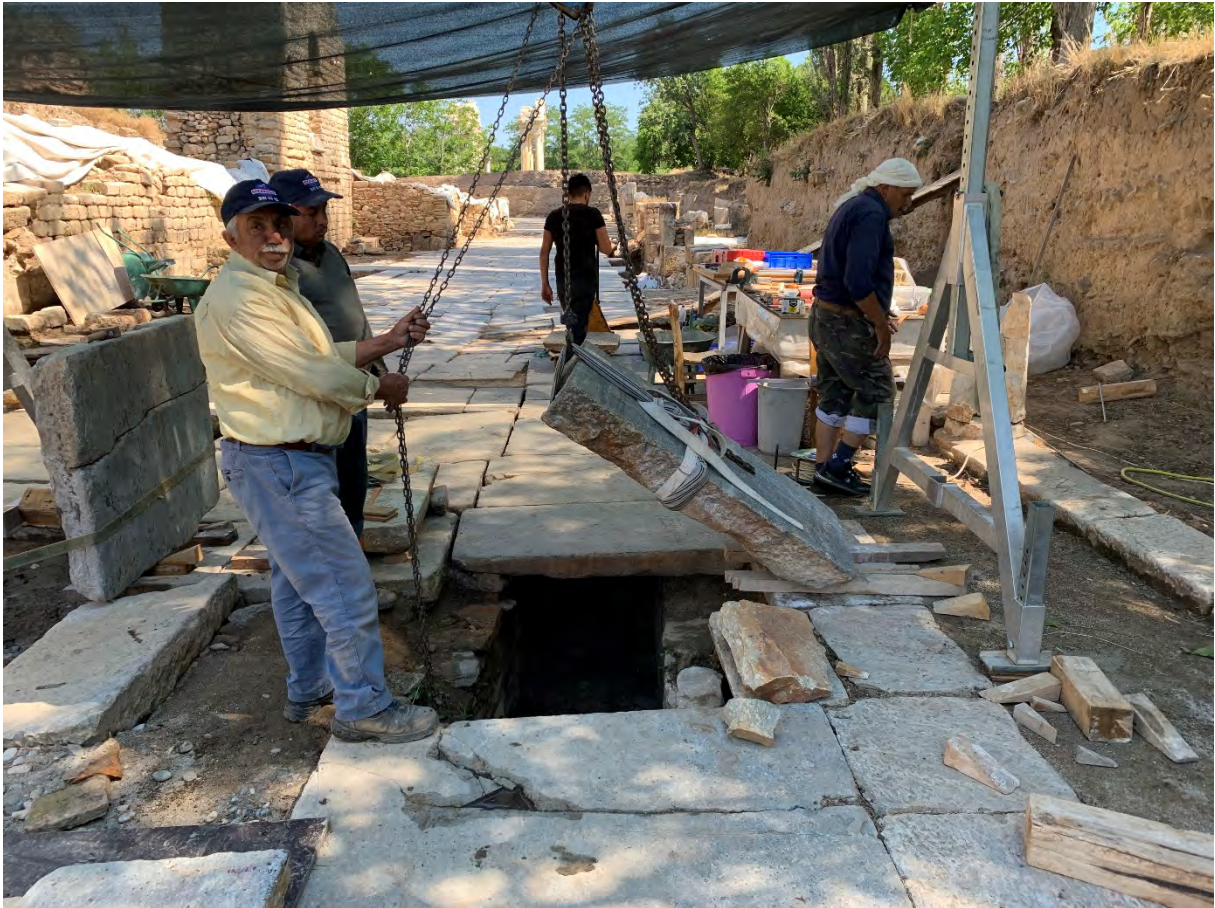
Figure 51: Site conservation. Repair of Tetrapylon Street paving (2022).
