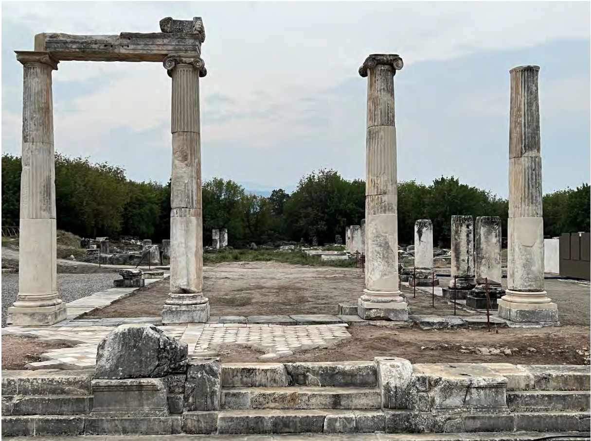
Figure 12: Civil Basilica. Anastylosis of colossal columnar order of vestibule (2022).
