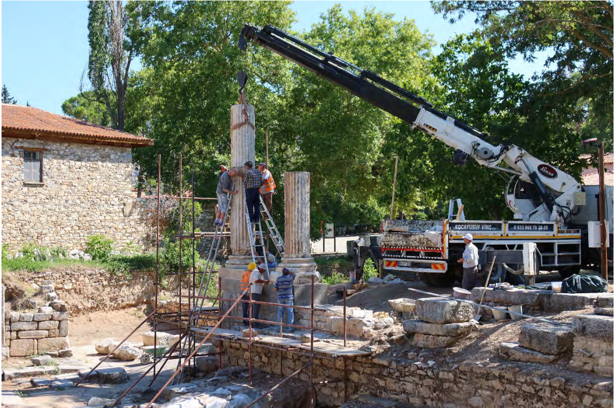
Figure 42: Sebasteion Temple. Anastylosis work on columns of temple façade, looking north-east (2022).
