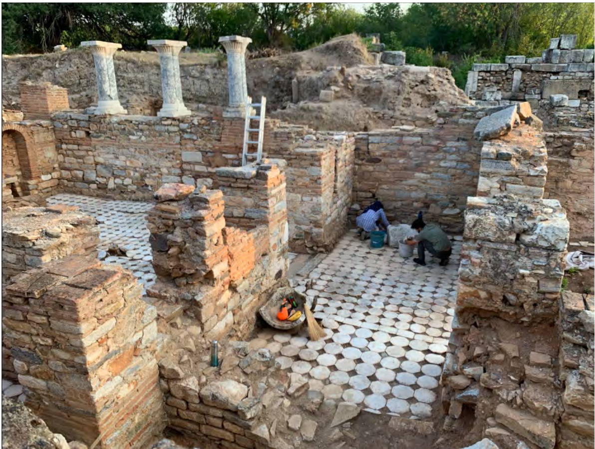
Figure 36: House of Kybele. Conservation work on tiled marble floor of Room 2, looking north (2022).
