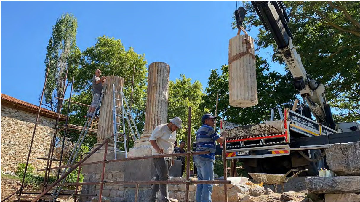
Figure 43: Sebasteion Temple. Anastylosis work on columns of temple facade (2022).
