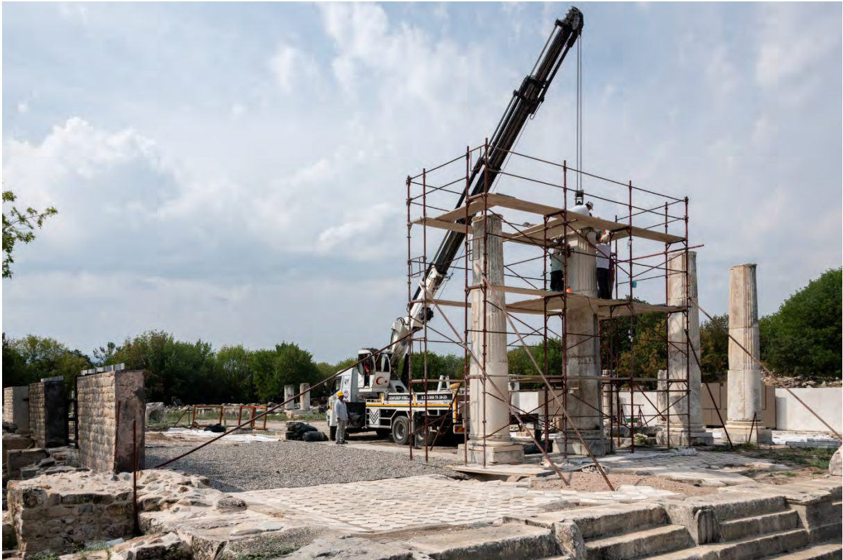
Figure 10: Civil Basilica. Anastylosis work in progress on colossal double-half-columns of vestibule (2022).
