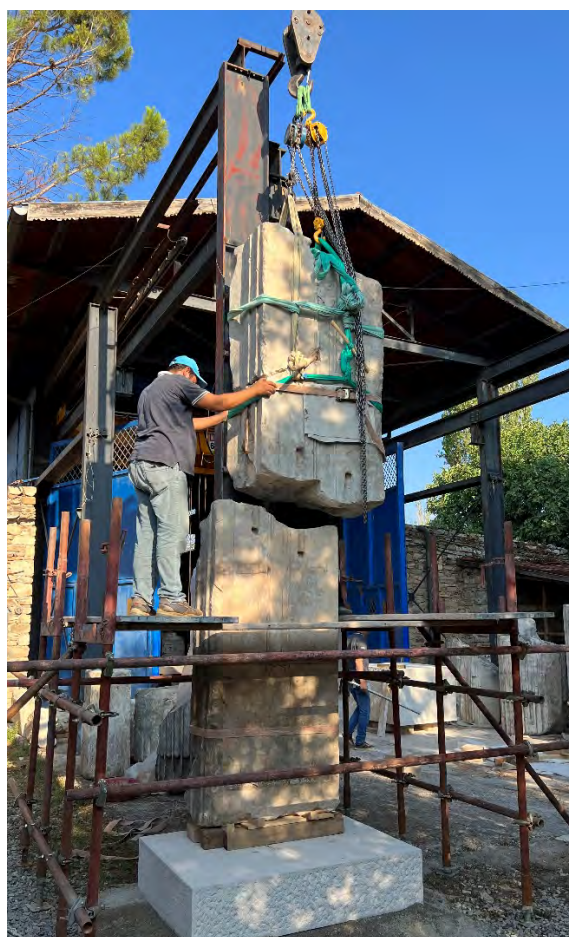
Figure 9A–B: Civil Basilica. A: Joining broken architrave. B: Hand-working flutes of replacement column drum (2022).
