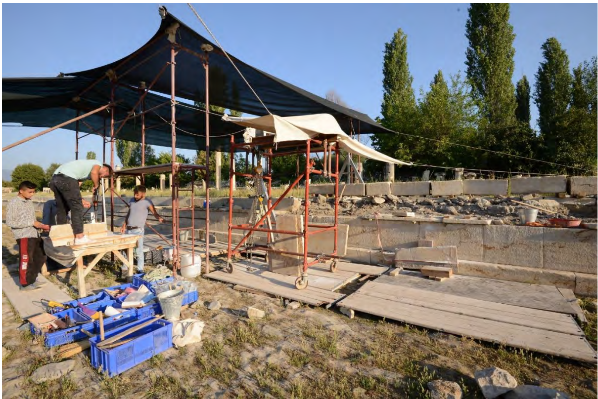
Figure 20: South Agora / Place of Palms. Conservation of pool perimeter, south side (2019).
