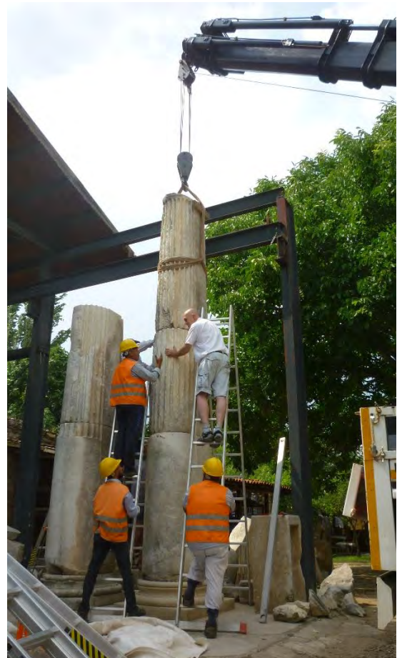
Figure 15: Basilica. (a) Hand-carving missing part of column in artificial stone. (b) Testing connection of column drums.
