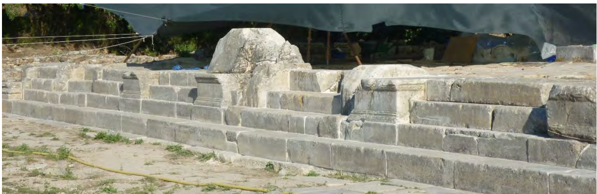
Figure 14a-b: Stepped entrance to Basilica façade, during and after conservation (2019).
