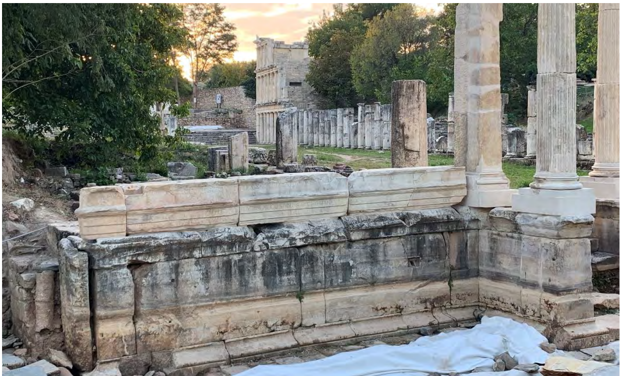
Figure 80: Complete surviving architrave-friezes from west end of Sebasteion's North Building, conserved and set in position on west podium of North Building (2019).
