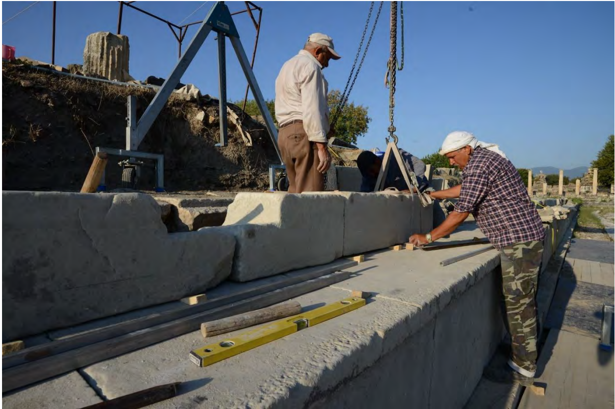
Figure 23: South Agora / Place of Palms. Conservation of inner seat blocks of pool perimeter, south side (2019).
