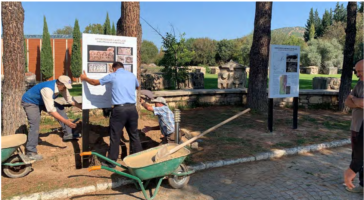
Figure 82: Installing two new visitor information signs about sarcophagi and marble quarries (2019).
