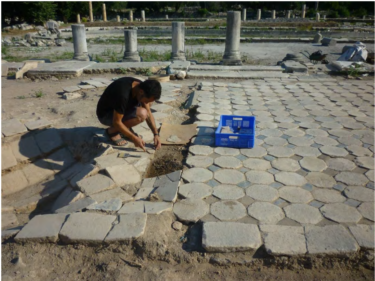
Figure 10: Basilica. Restoration of marble-tiled floor in Vestibule (2019).
