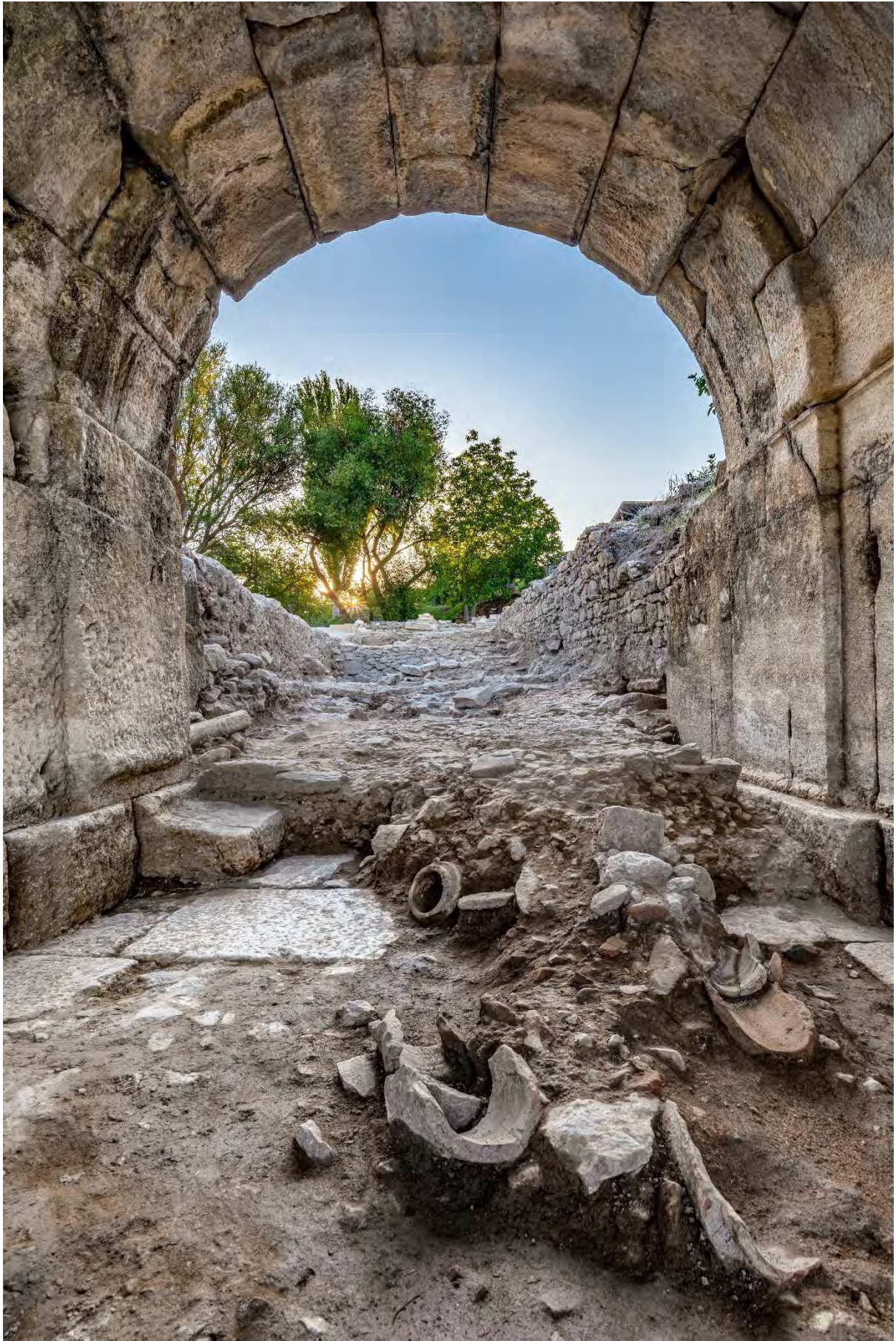
Figure 28: Tunnel under Agora Gate and ramp leading up to Street, view from west (2019).
