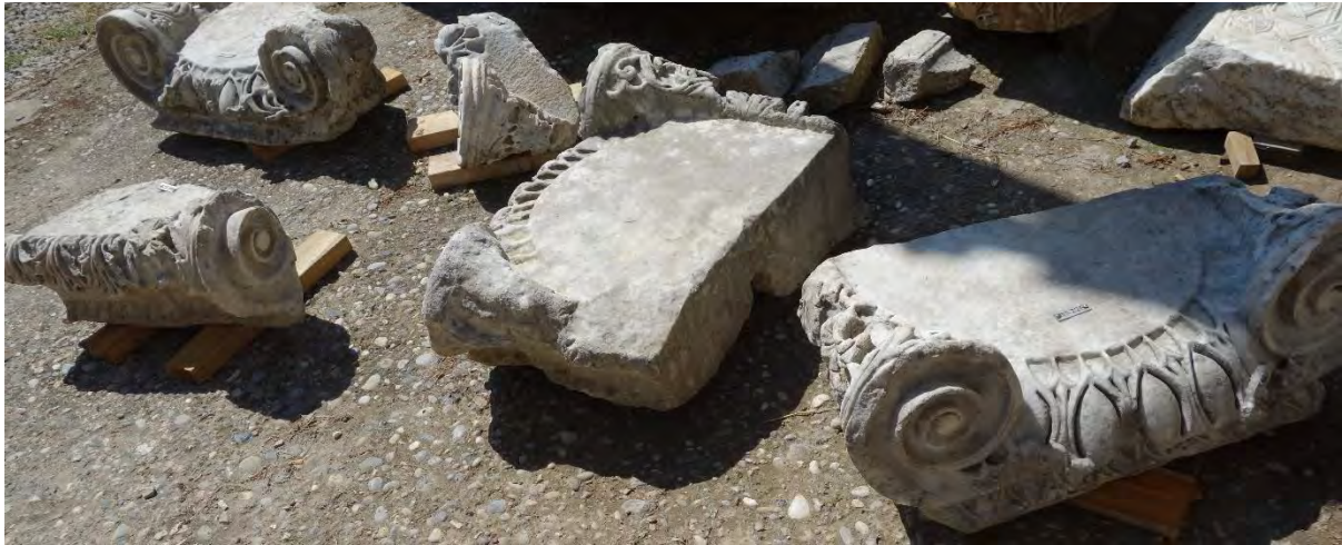
Fig. 36: Basilica. Broken Ionic capitals awaiting repair (2018).
