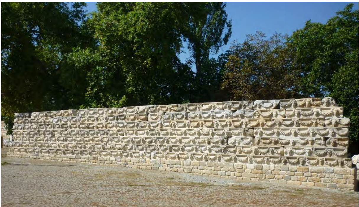
Fig. 51: Frieze Wall. Completed wall of mask-and-garland frieze blocks returned from Izmir to Aphrodisias in 2009 (2018).
