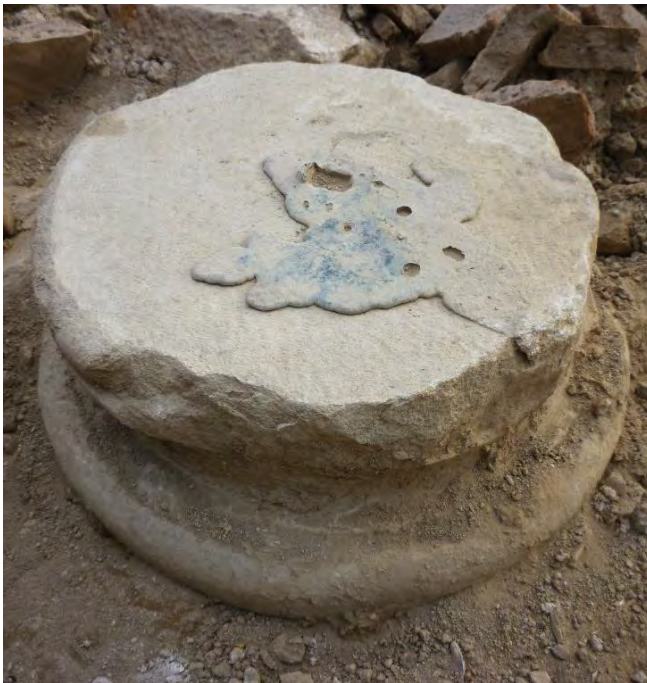
Fig. 7: Tetrapylon Street. Top of column base with poured lead for levelling column when placed on top of it. Fig. 8: Tetrapylon Street. Painted inscription on column invoking Emperor as 'lord of the inhabited world' (I 18-29 d)(2018).
