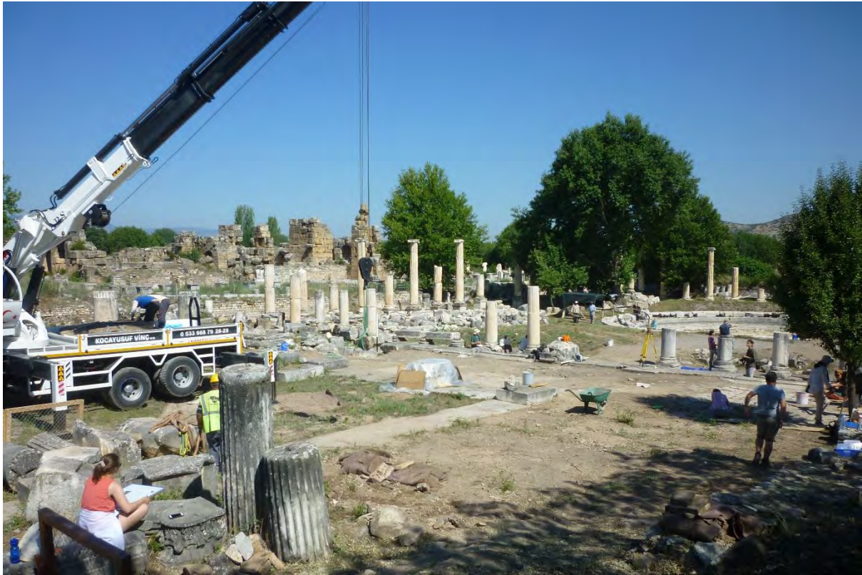
Fig. 33: Basilica. Moving of numbered blocks from north end of building (2018).
