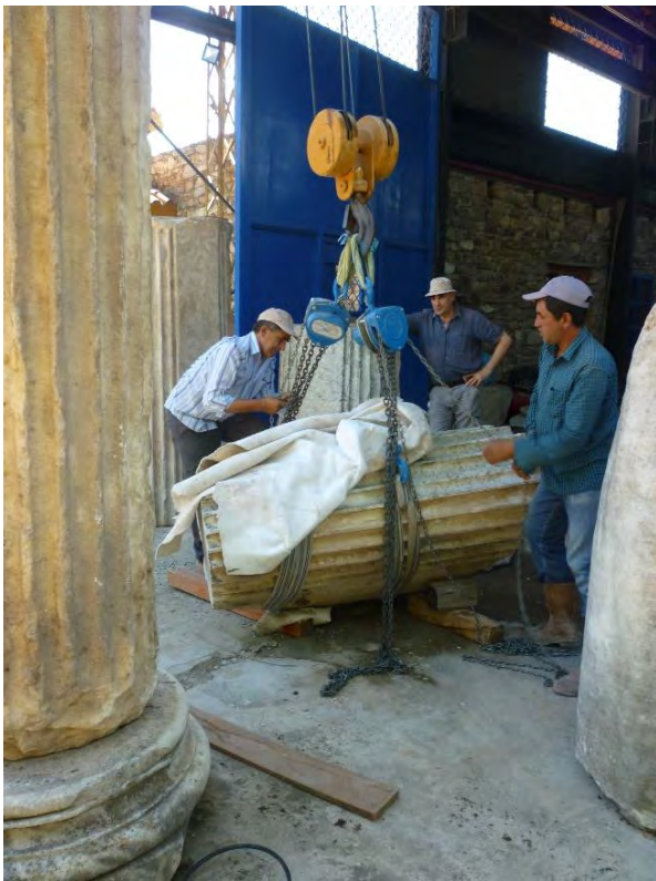
Figs. 34 - 35: Basilica. Moving and trial setting up of double half-columns from facade at conservation workshop (Blue Depot) (2018).
