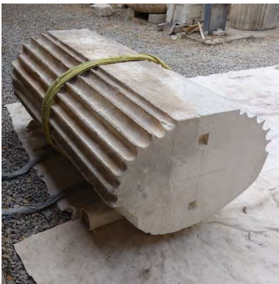
Figs. 39 - 40: Basilica. Column drum and base of double half-column completed with hand-carved artificial stone (2018).
