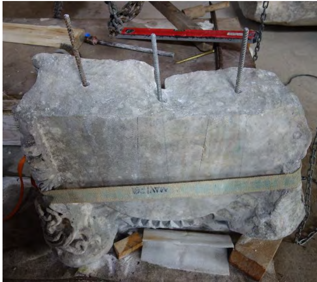
Figs. 37 - 38: Basilica. Doweling of broken Ionic capital of double half-column (2018).
