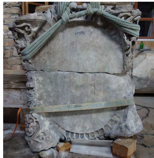
Figs. 37 - 38: Basilica. Doweling of broken Ionic capital of double half-column (2018).
