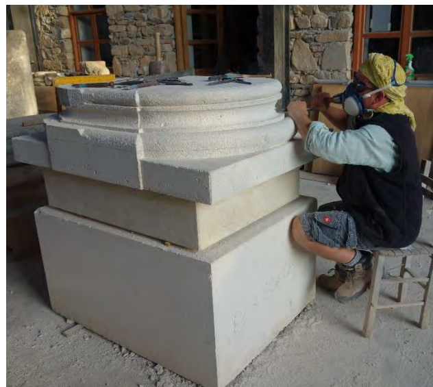
Figs. 39 - 40: Basilica. Column drum and base of double half-column completed with hand-carved artificial stone (2018).
