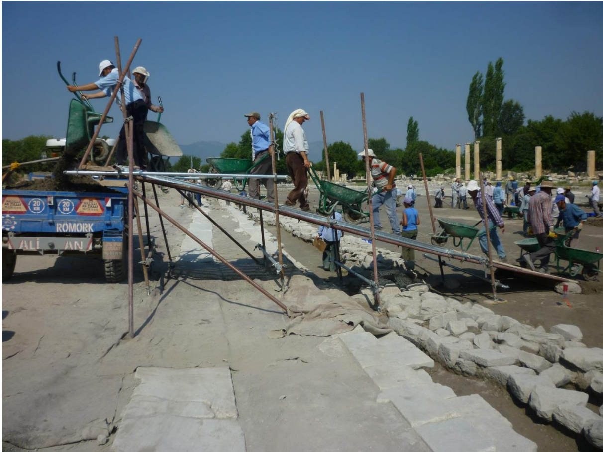
Fig. 5: Steel ramp for removing excavated earth from pool (2017).
