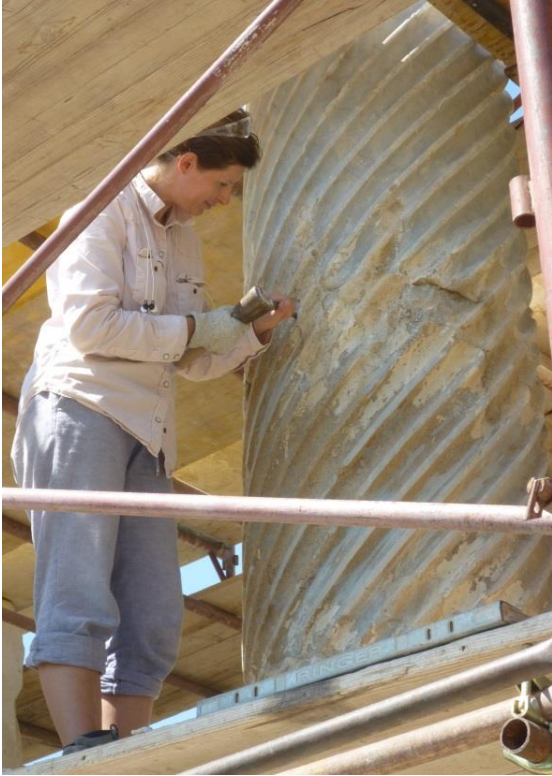
Fig. 46: Joanna Skwierz of Cliveden Conservation restoring spiral flutes of column on east side of Tetrasyon. Fig. 47: Restored paving slabs of late antique street (2017).
