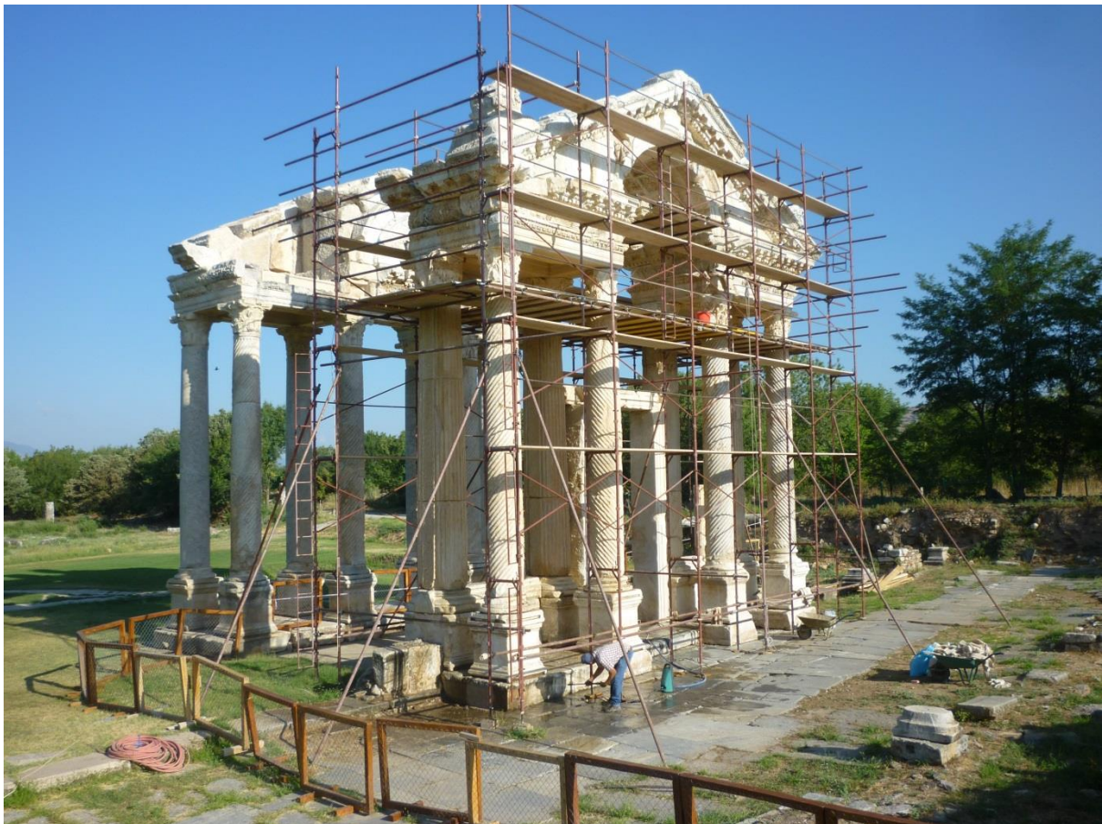
Fig. 45: Scaffolding and conservation work on east side of Tetrapylon (2017).
