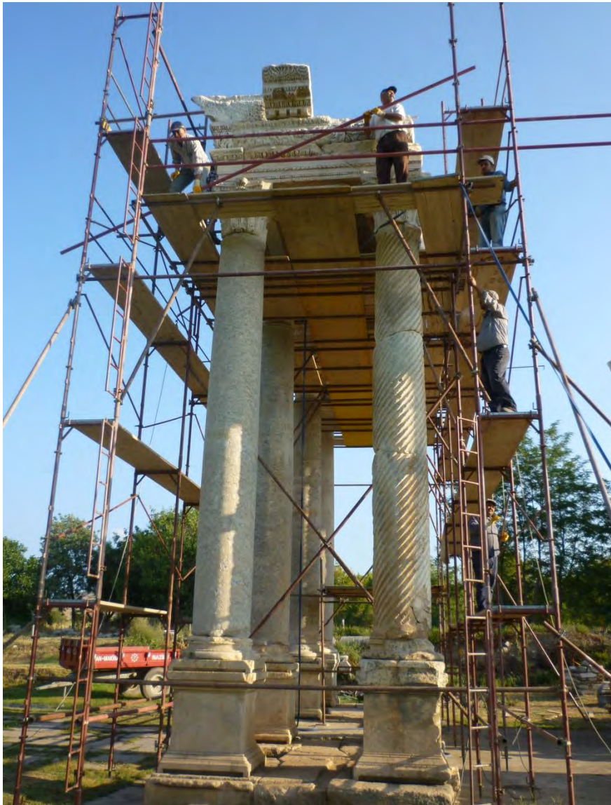
Fig. 28: Tetrapylon, conservation and maintenance work (2016).
