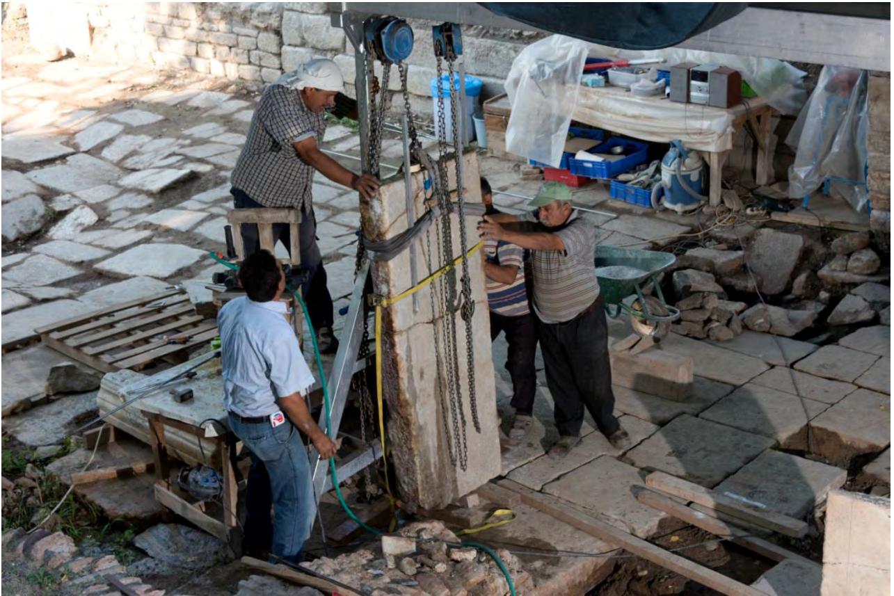
Fig. 23: Tetracylon Street, conservation of paving and drain covers (2016).
