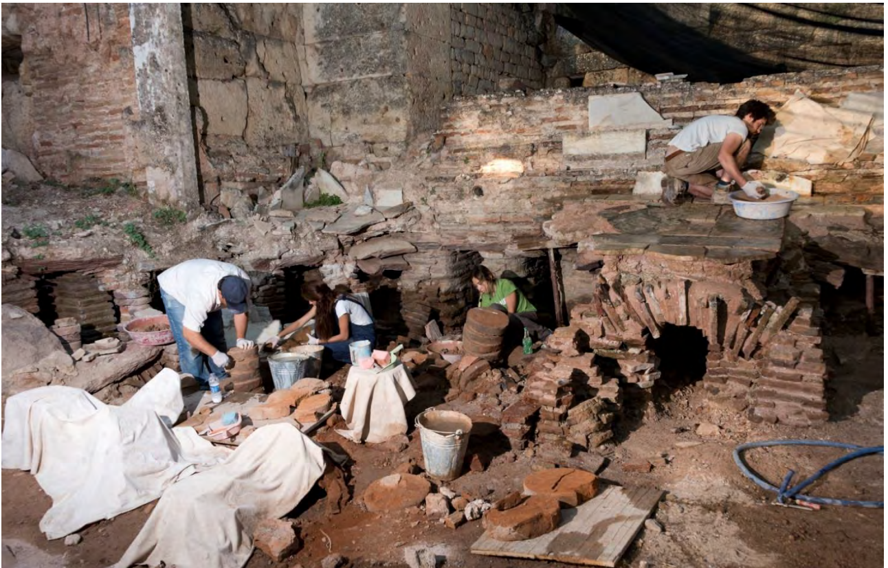
Fig. 17: Hadrianic Baths, Room 4, conservation work in progress (2016).
