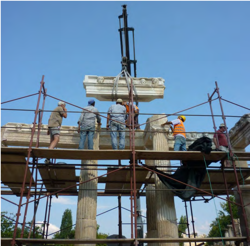
Figure 20: Sebasteion Propylon. Anastylosis: architrave-frieze block is craned into position (2015).
