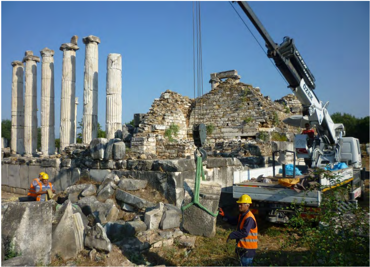
Figure 28: Temple-Church: moving of blocks from south-east corner of building (2015).
