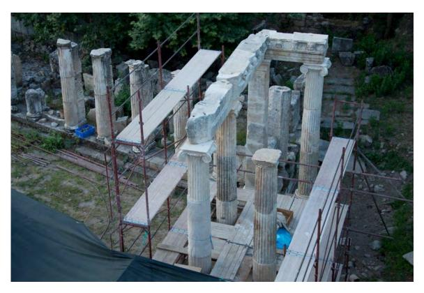
Fig. 7: Sebasteion Propylon, anastylosis, columns and architrave-friezes (2014).
