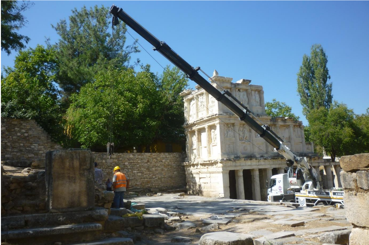
Fig. 43: Sebasteion Temple. Restoration work on front of temple (looking southwest) (2021).
