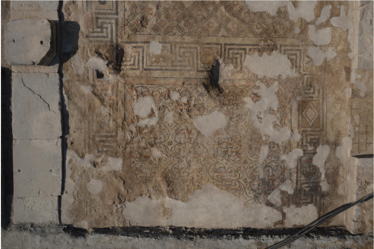
Fig. 4: Civil Basilica, part of east aisle mosaic floor (AD 350s) excavated in 2021.
